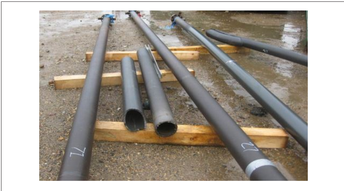
Fig. 3. Damaged reformer tubes
